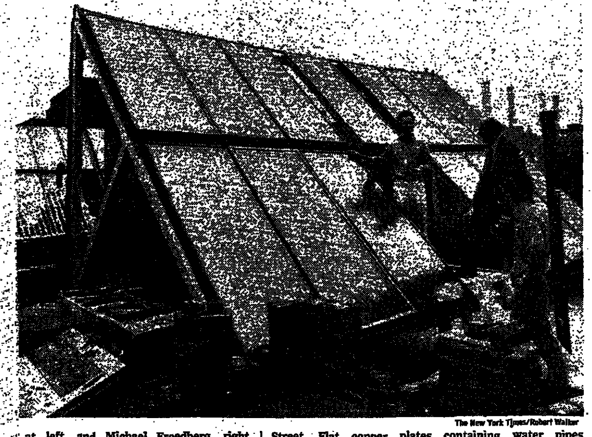
at left, and Michael Freedberg, right, stative Edward I. Koch the solar energy alled on the roof of 519 East 11th Street. Flat copper plates containing water pipes are tilted toward the sun; the system provides for 85 percent of the building's hot water requirements.
